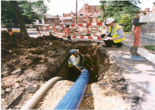
Testing pipelines for water utilities
